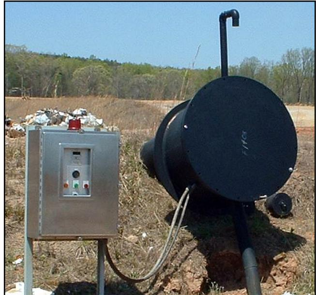
LEACHATOR control panels come standard with a window kit so operators can view system status without opening the enclosure.
